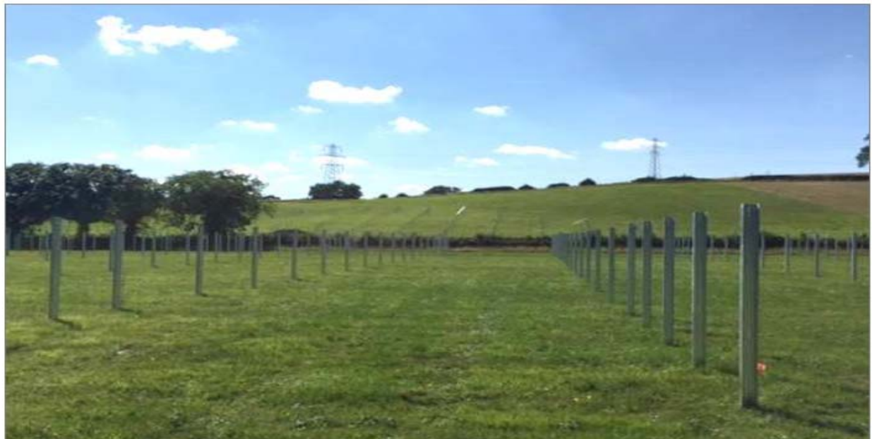
Figure 9 – Example of Piles for a solar farm in place
